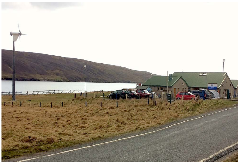
Above: A small scale wind turbine in a domestic setting in Shetland. The small scale of the turbine allows it to fit unobtrusively into the surrounding landscape. © Pete Bevington/www.shetnews.co.uk
