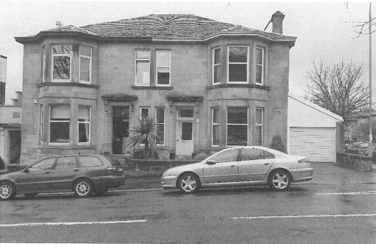
2. View from Forsyth Street, no panels visible at all.
